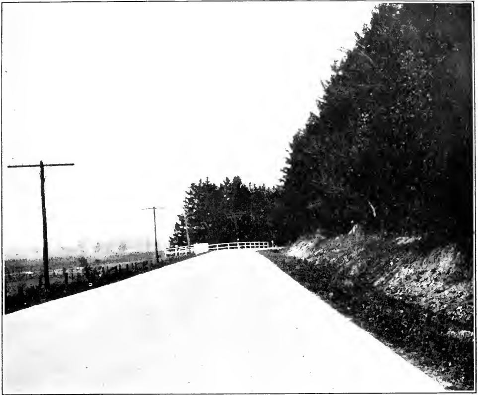
HAMILTON-GUELPH PROVINCIAL HIGHWAY Cement concrete surface 20 feet wide, south of Guelph.
